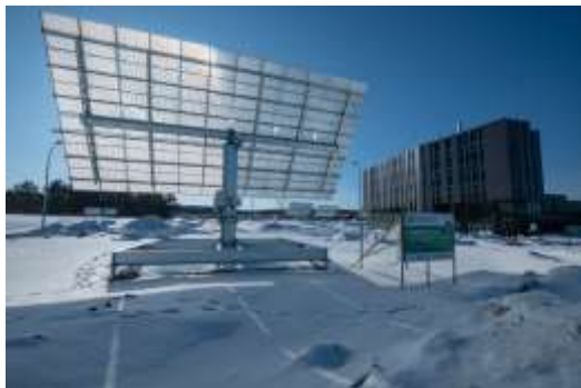
Figure 1. Picture of a commercial 12 modules concentrated photovoltaic system installed at Université de Sherbrooke. It embeds 14,400 couples of Fresnel lens /solar cell with an optical concentration \sim 500\times .
